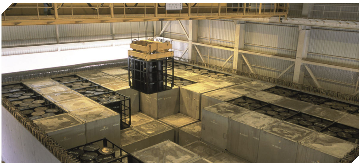
Image of the filling of a LILW disposal vault.
