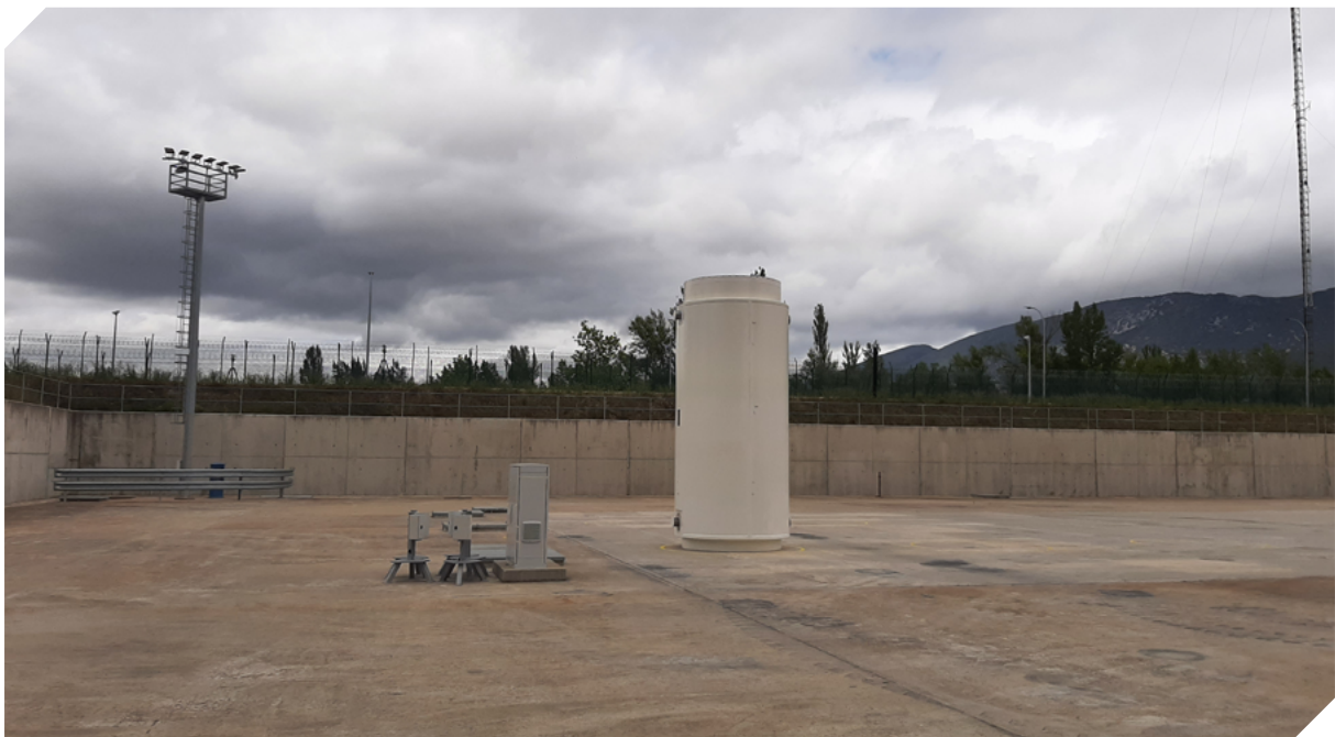
General view of the Santa María de Garoña Nuclear Power Plant ITS.
