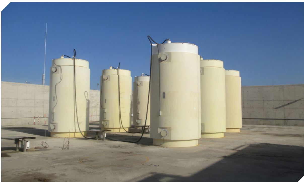
General view of the Almaraz Nuclear Power Plant ITS.
