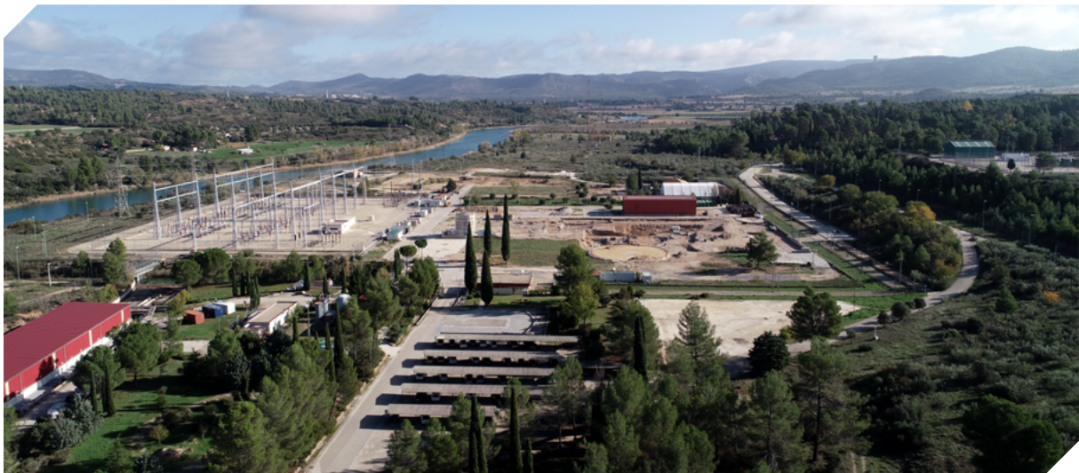
Picture of the decommissioning of José Cabrera Nuclear Power Plant.
