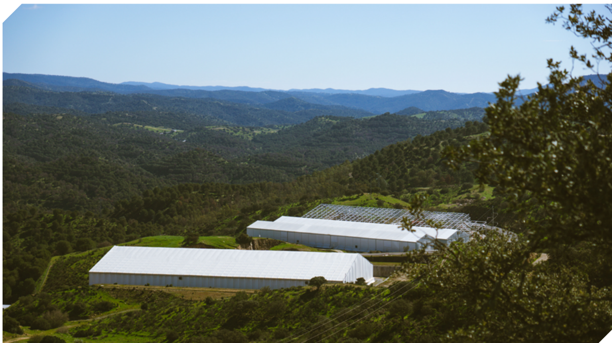
Image of the VLLW disposal vaults at El Cabil Disposal Facility.
