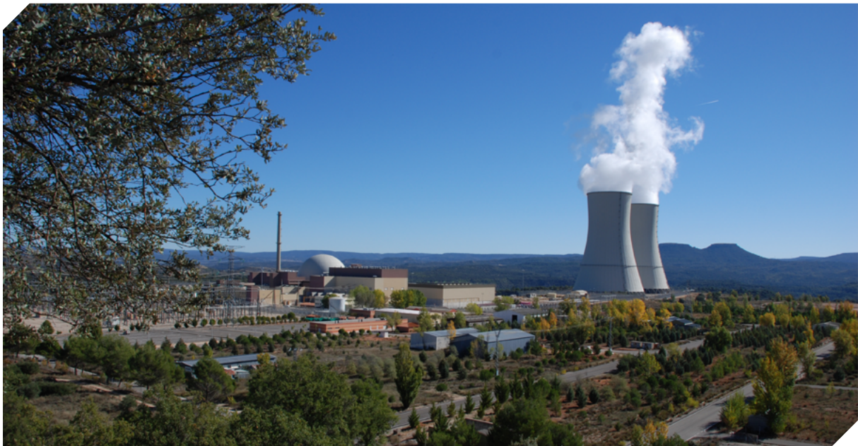
Overview of the Trillo Nuclear Power Plant.
